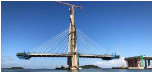
Figure 4. A cable stay bridge under construction
